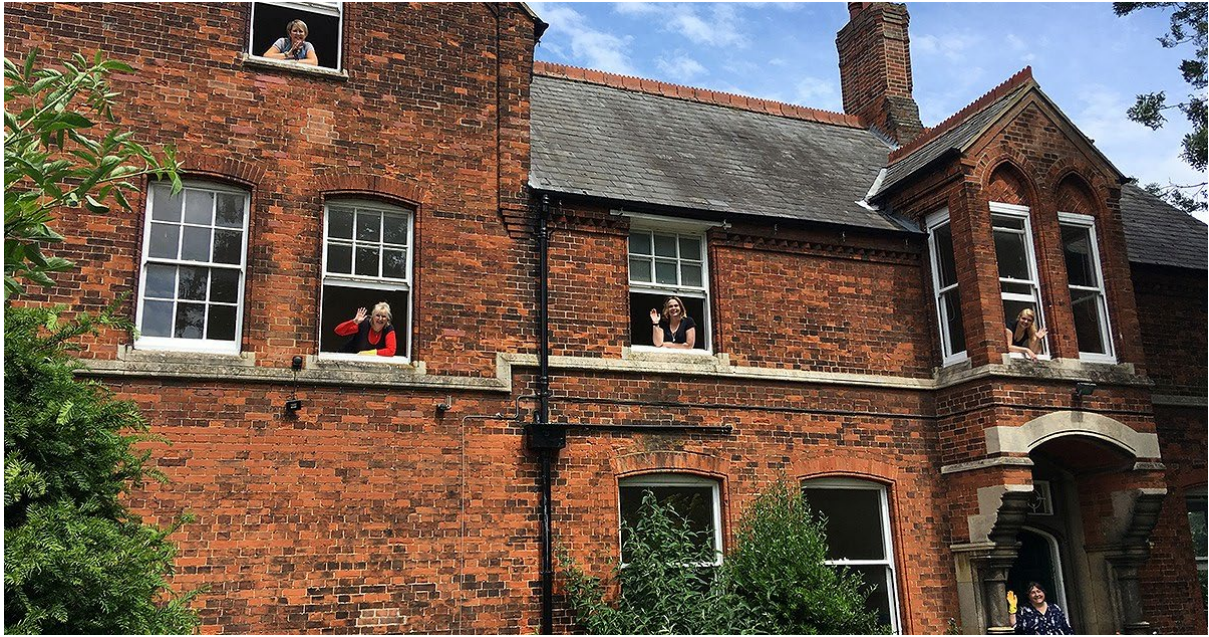
The new Winter Night Shelter building for the homeless which is being made ready for opening at the end of October 2020 for a 5-month season, 7 nights per week.
